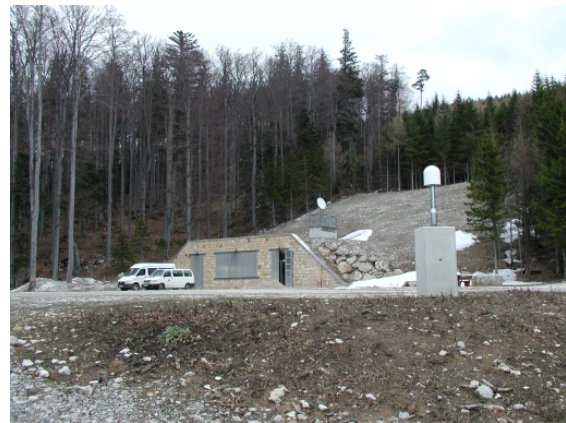
Figure 1: EPN/APOS GNSS-Antenna on a stable pillar/ concrete block in front of the observatory.
